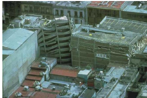
Figure 1.6 Waffle Slab Buildings at Mexico City after Earthquake Occurred in 1985 (johnmartin.com)
