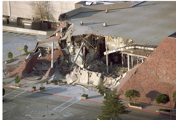
Figure 1.5 Bullock's Department Store after Collapse (deseret.com)
